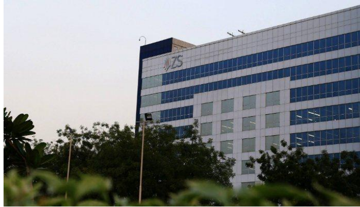
Fig. 1.1- ZS Associates Gurugram Office
