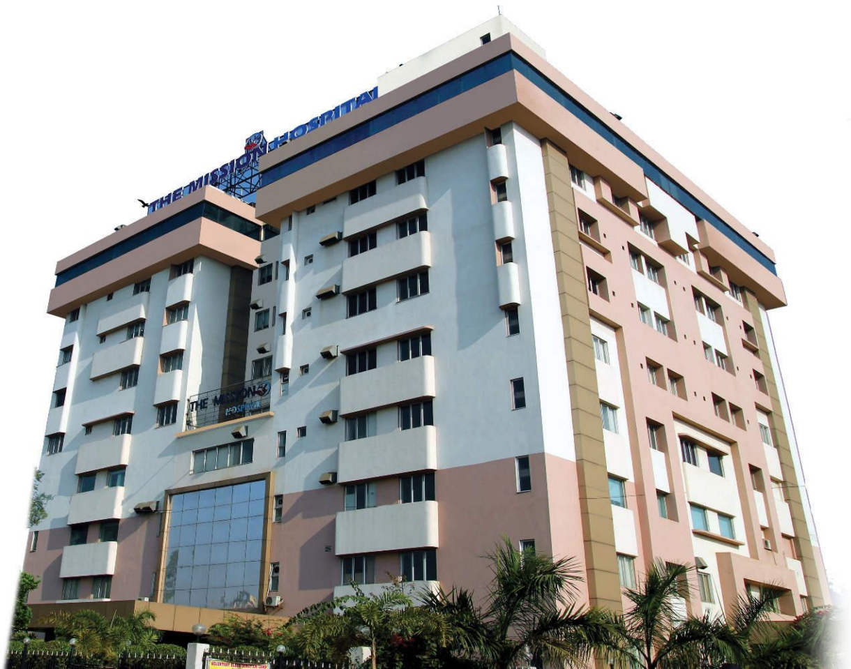
The Mission Hospital, Durgapur
