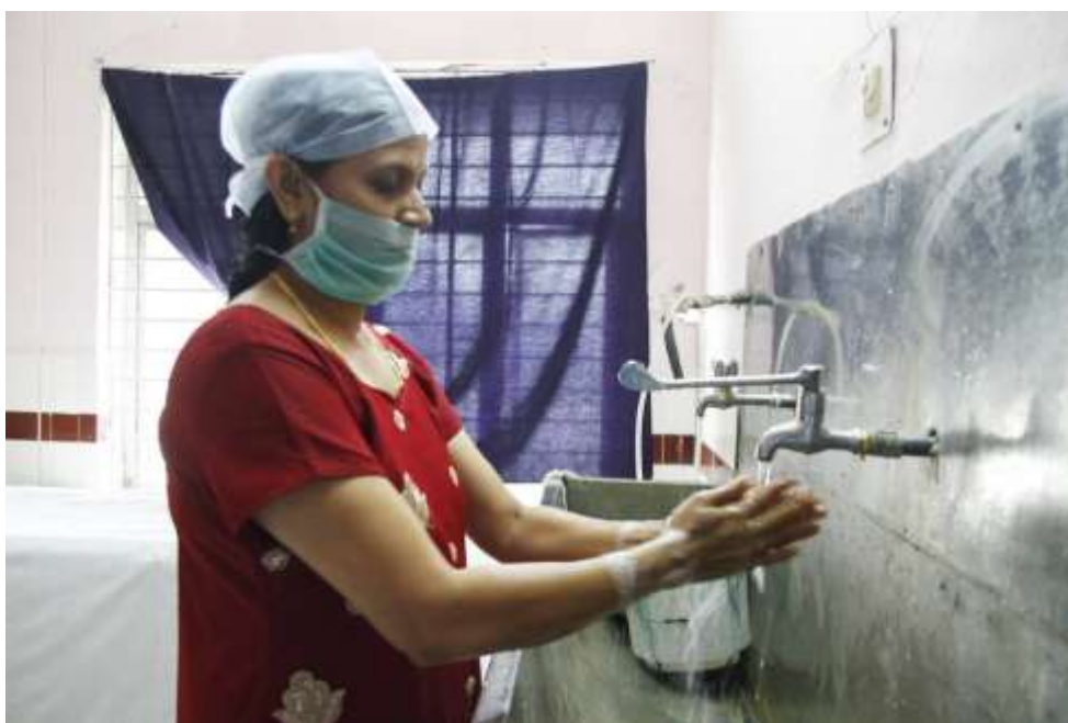
Figure 2.8. Figure showing the elbow operated tap used a healthcare personnel
