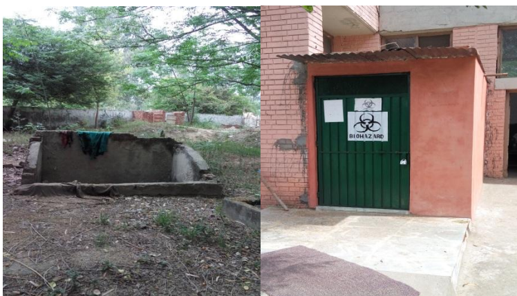
Fig.4 BMW storage area (before) and BMW store room kept in lock (after)
