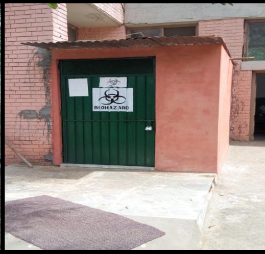
BMW store room kept in lock (after)
