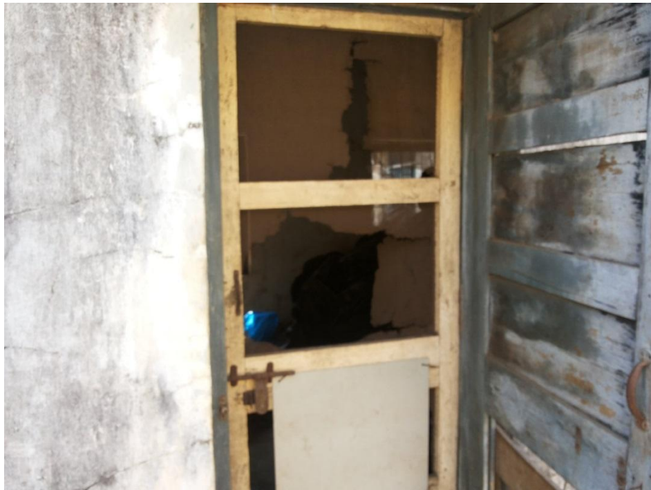
Figure 3: Door of the BMW storage Room
