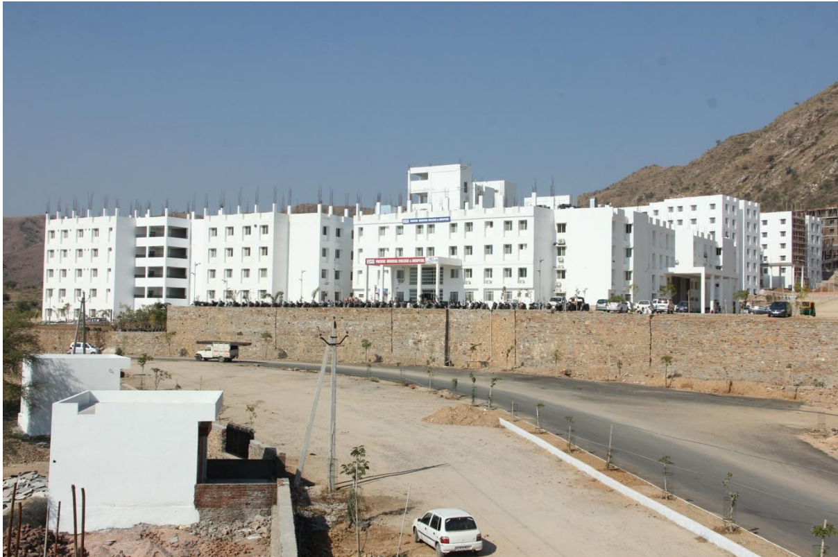
Figure 1 Multispecialty 402 Bedded hospital in Udaipur area catering to Udaipur , Abu road, Raj samand , Nathdwara,
