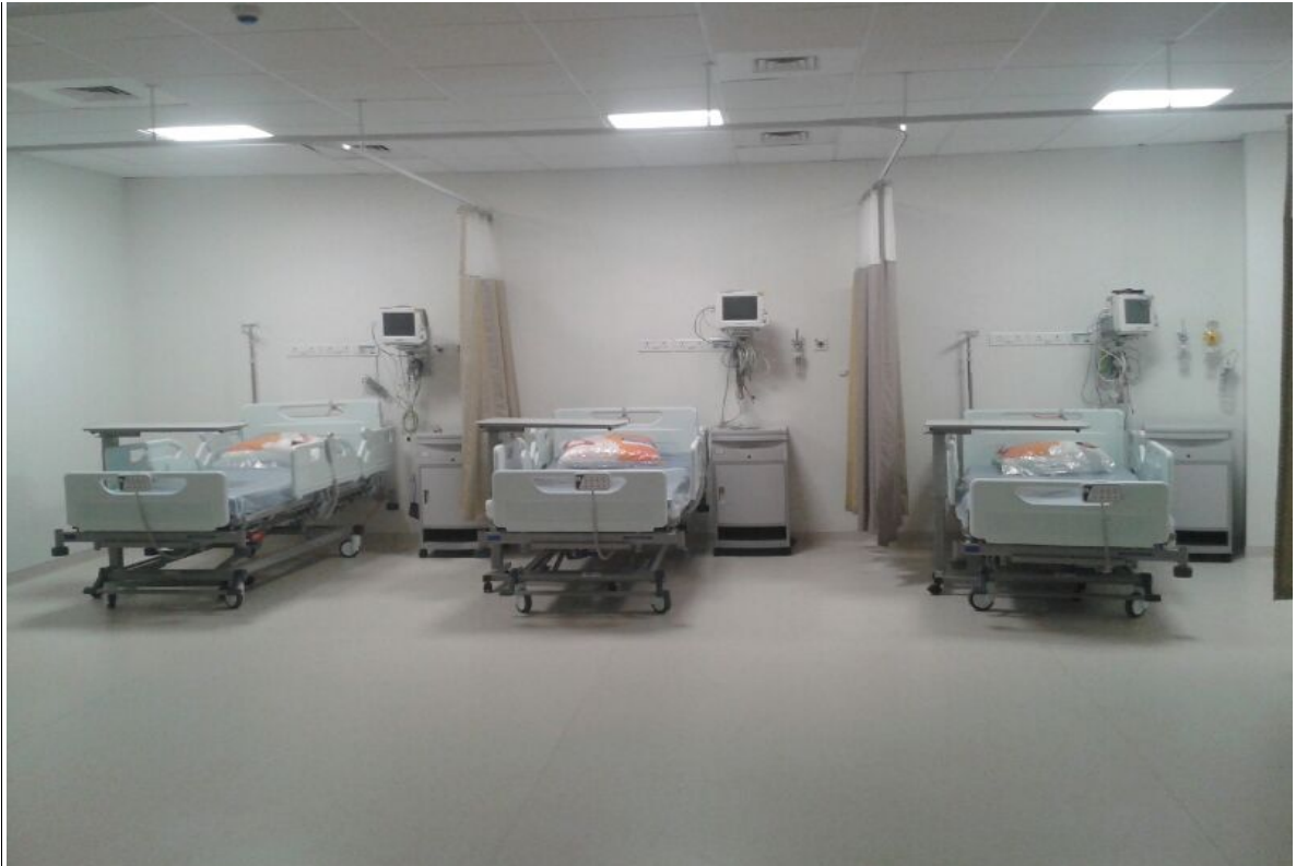
Image 11: Paediatric Bay after equipment installation
