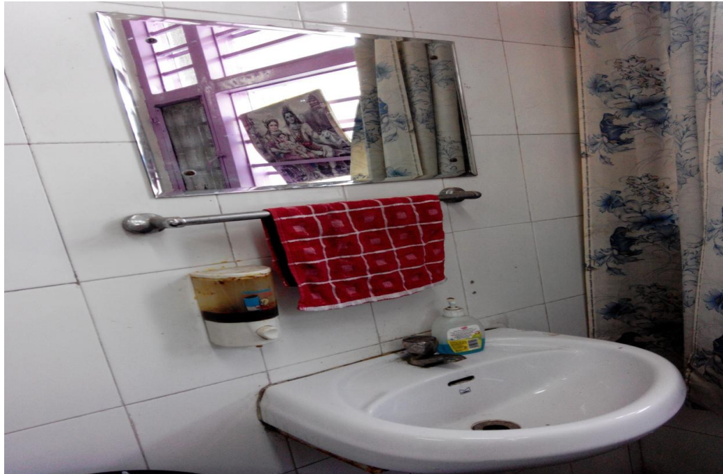
Wash basin, dispenser, towel rails and sanitizers in OPDs.
