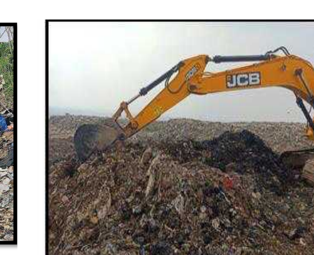
PHOTO SHOWING REMEDIATION WORK IN PROGRESS
