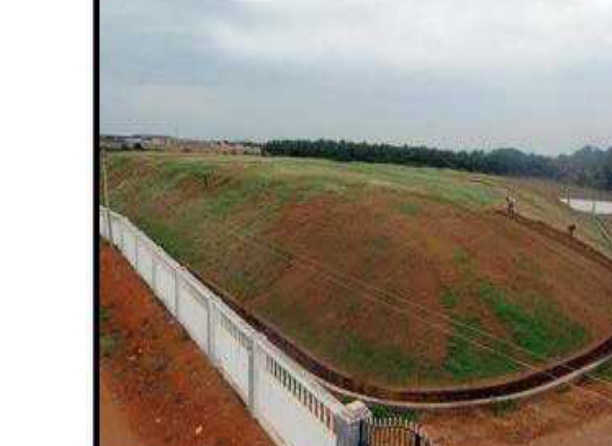
PHOTO SHOWING REMEDIATION WORK COMPLETED
