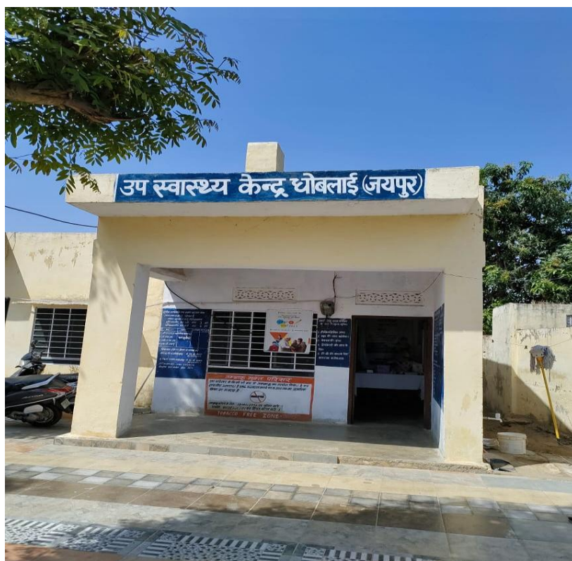
Fig10: One of the subcenter attached to the CHC open containers presents inside the facility.
