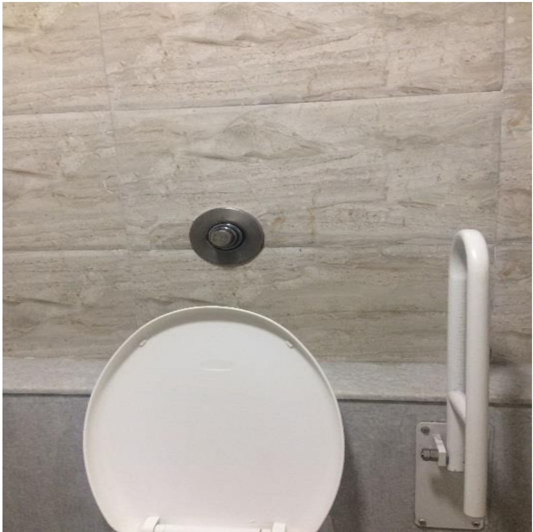
Grab bars installed
