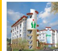
Fortis Hospital, Shalimar Bagh, New Delhi
