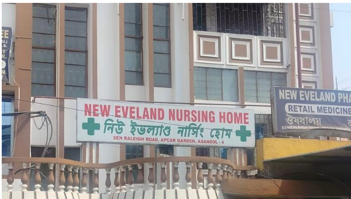
Fig. 10: New Eveland Nursing Home, Asansol
