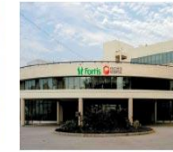
Fortis Escorts Hospital, Faridabad
