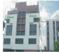
Fortis Malar Hospital, Chennai
