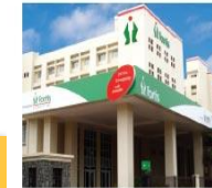
Hiranandani Fortis Hospital, Vashi, Mumbai
