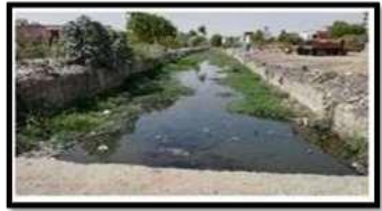
Fig. 3.11 Open drains at AIIMS Road
