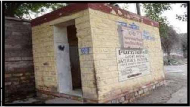
Fig.3.13 Public Toilet at Paota Circle
