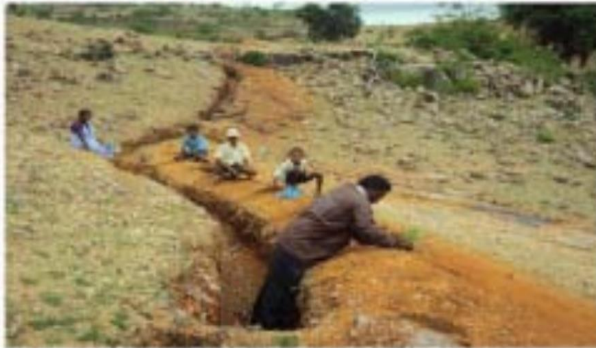
Ridge area treatment with CCT
