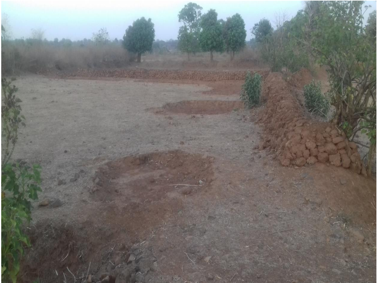
Med Bandhan work in private land of villagers
