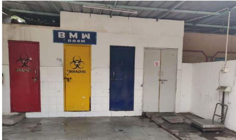
Fig 24: Biomedical Waste Room at BMCHRC
