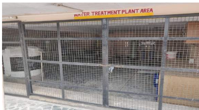
Fig 25: Water Treatment Plant at BMCHRC
