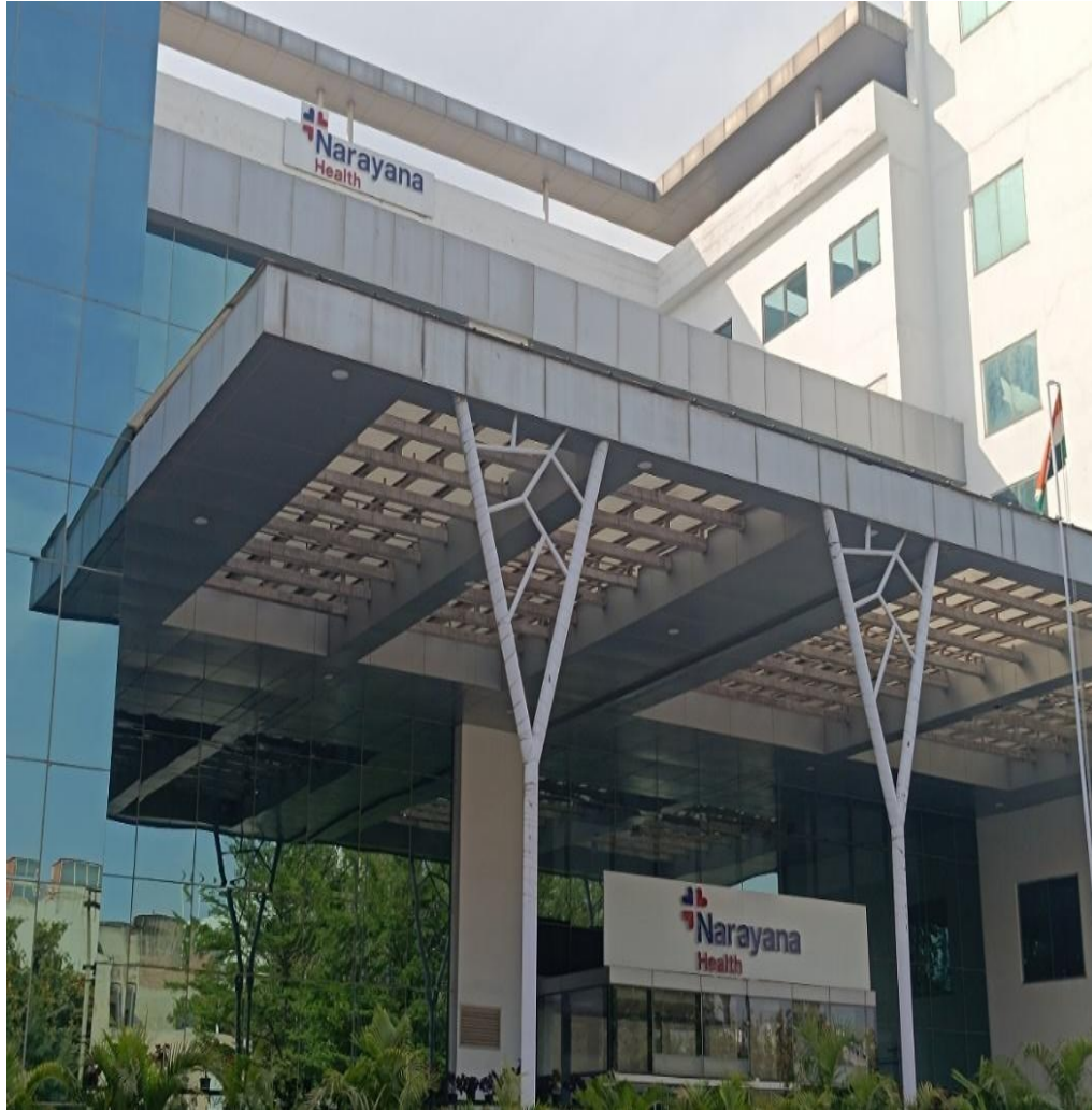
Fig 2. OPD Entrance of Narayana Hospital, Gurugram
