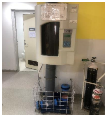
Figure 1.3- Pneumatic Tube station
