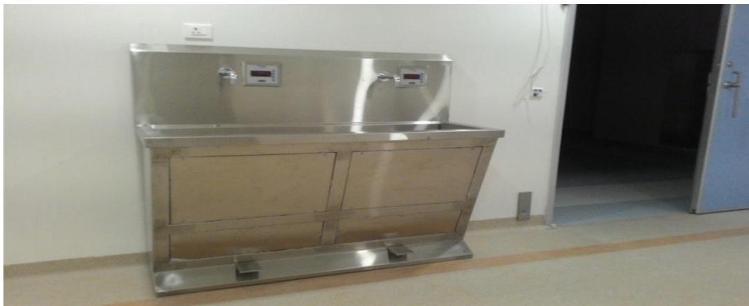
Fig.no.7.8 scrub sink sensor based
