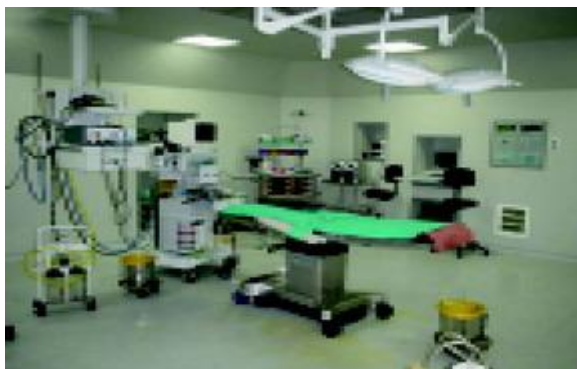
Fig.no. 3.1: An inside view of the Operating Room
