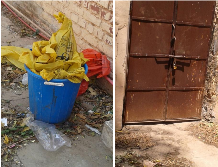
Backdoor of Labour room oened into open space area,used exclusively for carrying biomedical waste
