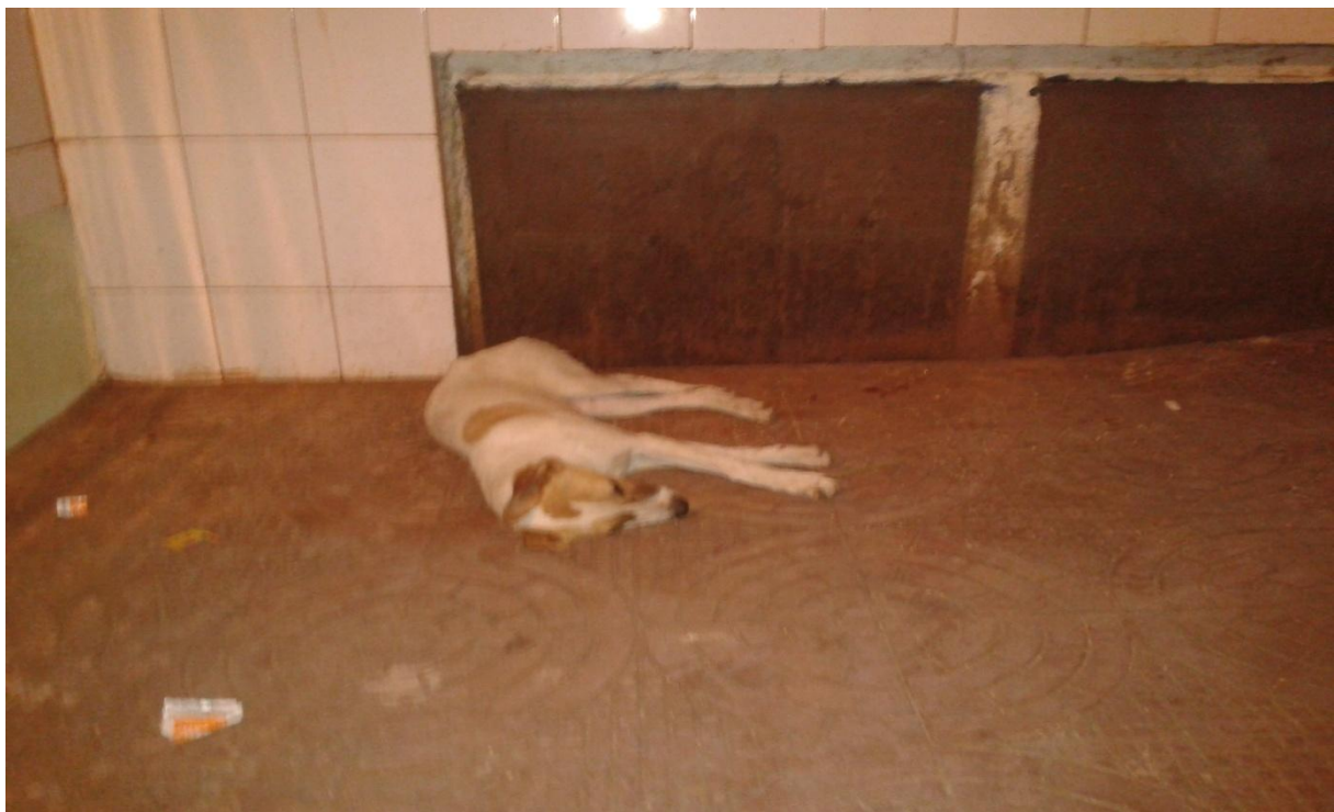
Figure 1: SNCU & Labour room connected by an unhygienic ramp
