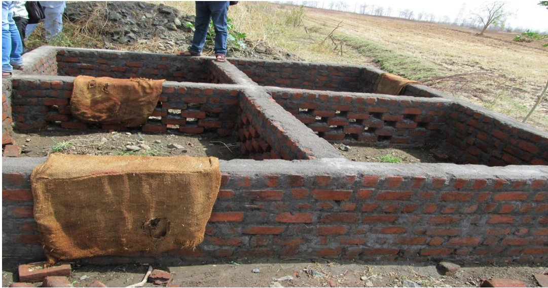
Four Pit Structure
