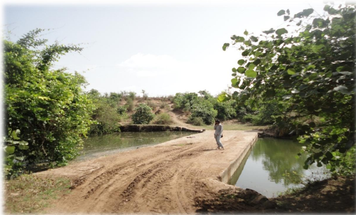
Picture 2: Existing watershed structure (Check dam cum cause way)
