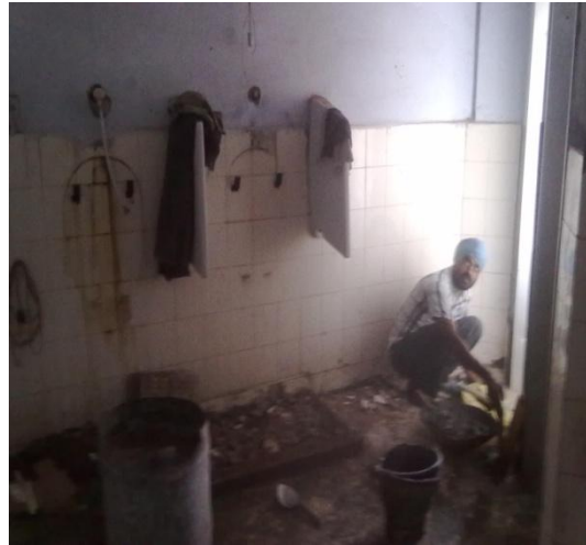
TOILETS (work in progress.)
