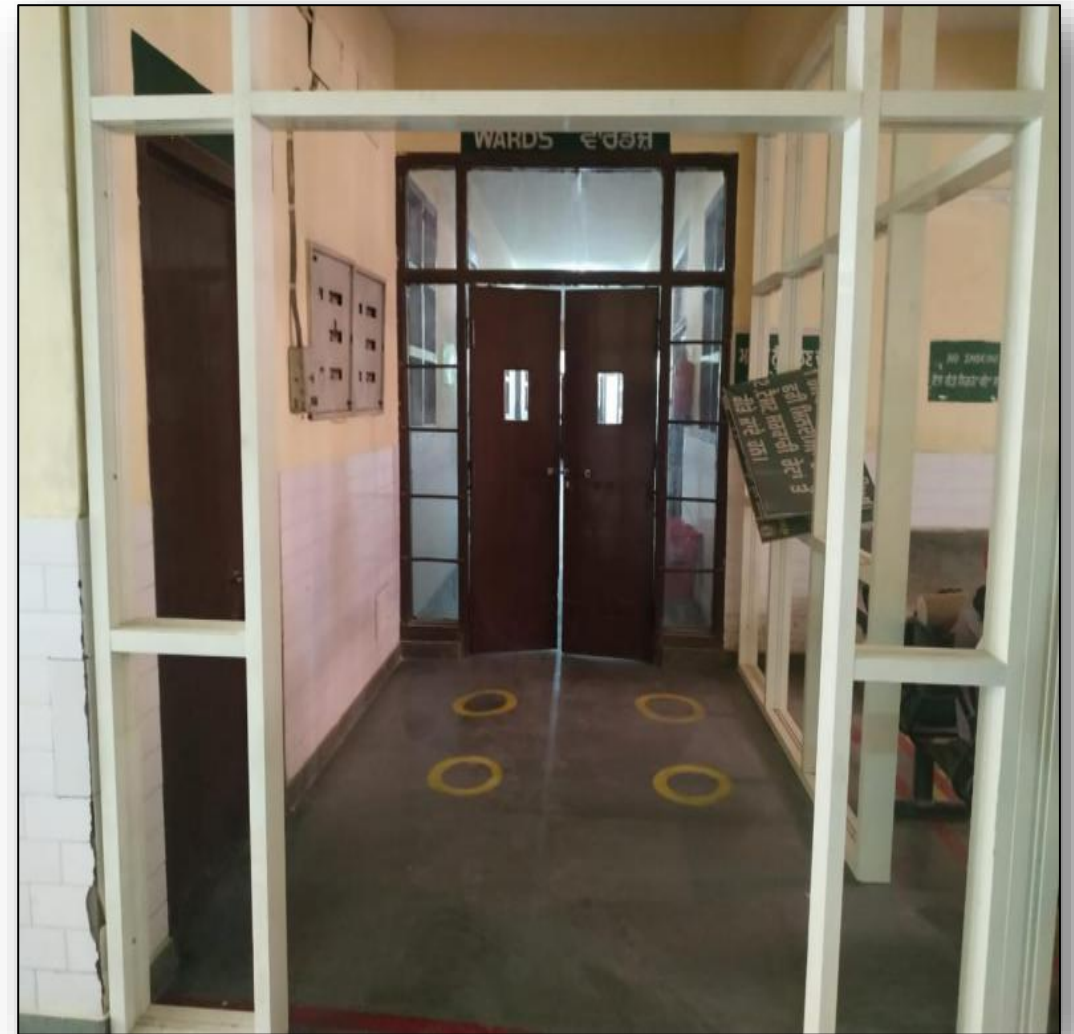
Dedicated donning and doffing area under construction at S.D.H BATALA.
