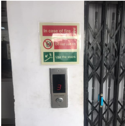
Fig- in case of fire signage
